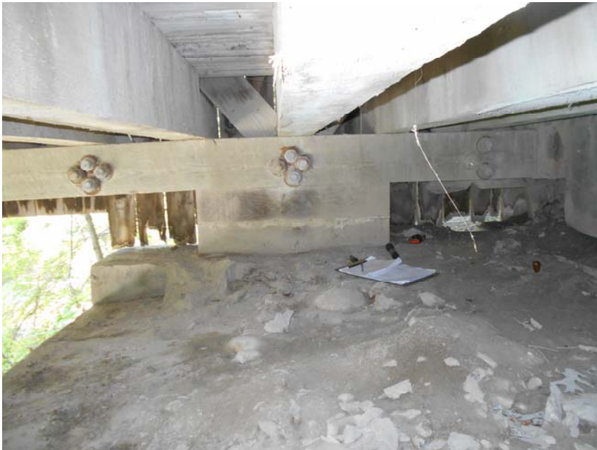
Existing Bearing Blocks
